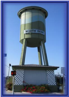
AT&T Faux Water Tank Antenna Installation
